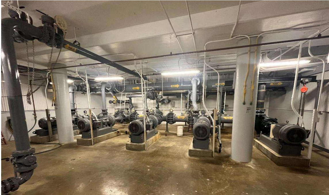
FIGURE 3-4: RETURN ACTIVATED SLUDGE PUMP GALLERY
