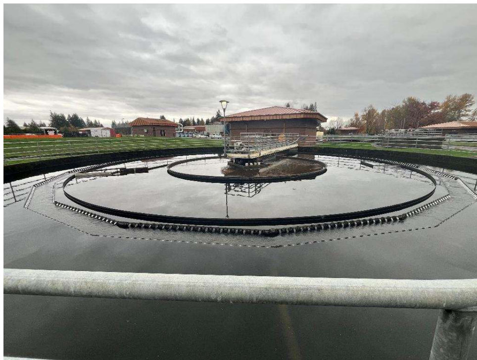
FIGURE 2-2: CLARIFIER 2 UNDER STRESSED CONDITIONS
