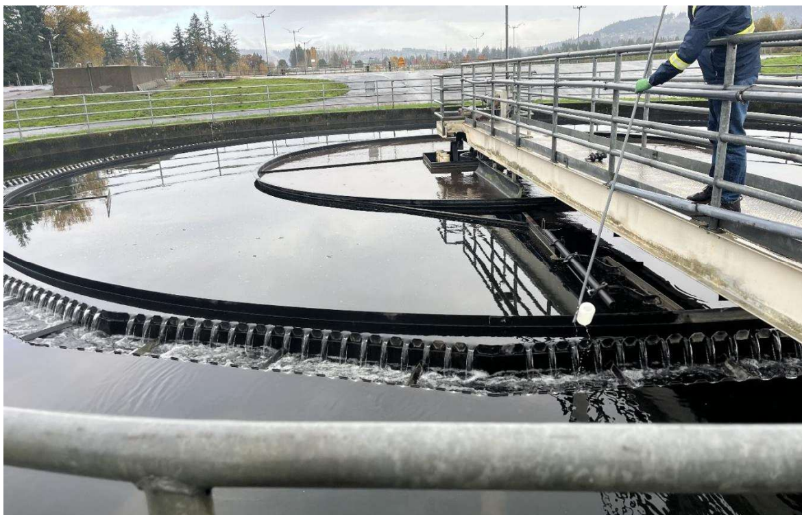
FIGURE 2-1: CLARIFIER SAMPLE COLLECTION AT CLARIFIER 2
