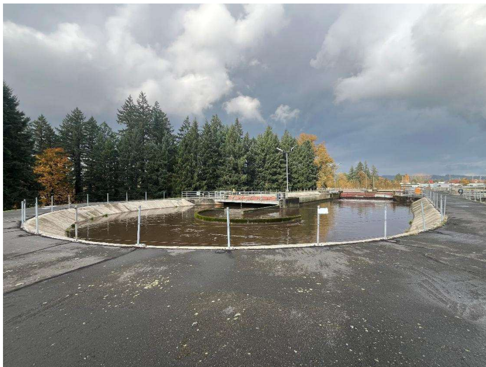
FIGURE 2-3: OXIDATION DITCH DURING STRESS TESTING
